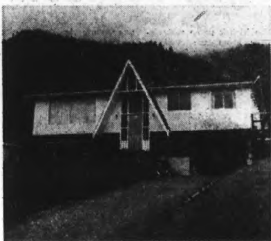
NEW HOUSES such as this one have replaced old camp homes at Sayward where forest workers can have comforts of city life while working in bush.
